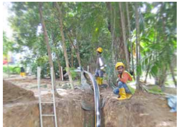
Figure 2: The SureFIT® winds its way to the construction pit.
