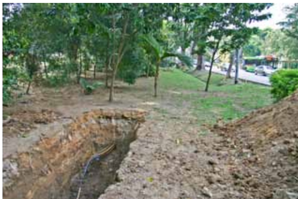
Figure 1: Laying of SureFIT®-Liners with unhindered traffic and minimal earthworks.
